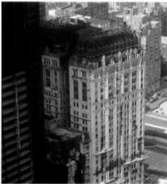
The Moinian Group is currently in the process of applying for $100 million in Liberty Bonds to convert the 36-story New York Athletic Club at 18 West St. into 288 residential apartments.
